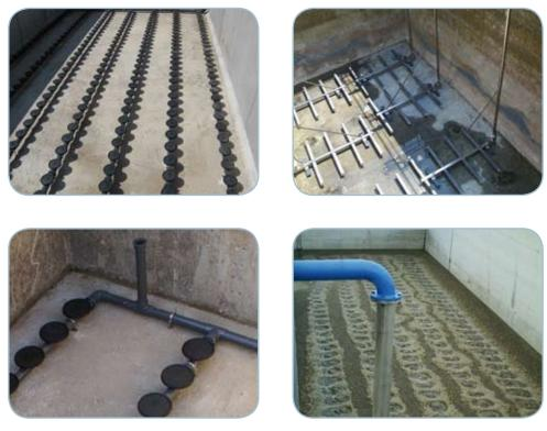
The Zenit range includes both disc and tube membrane air diffusers.
